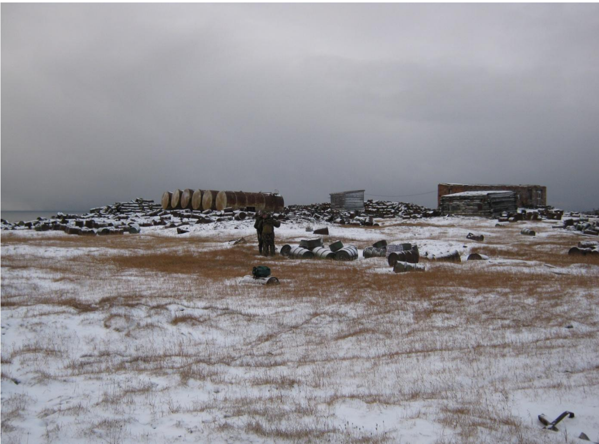
Figure 37. Tanks Near Diesel Station on Bolshoi Liakhovsky Island
