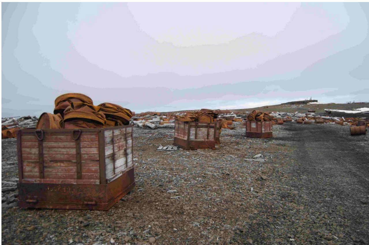
Figure 23. Fuel Drums Pressed and Prepared for Transportation
