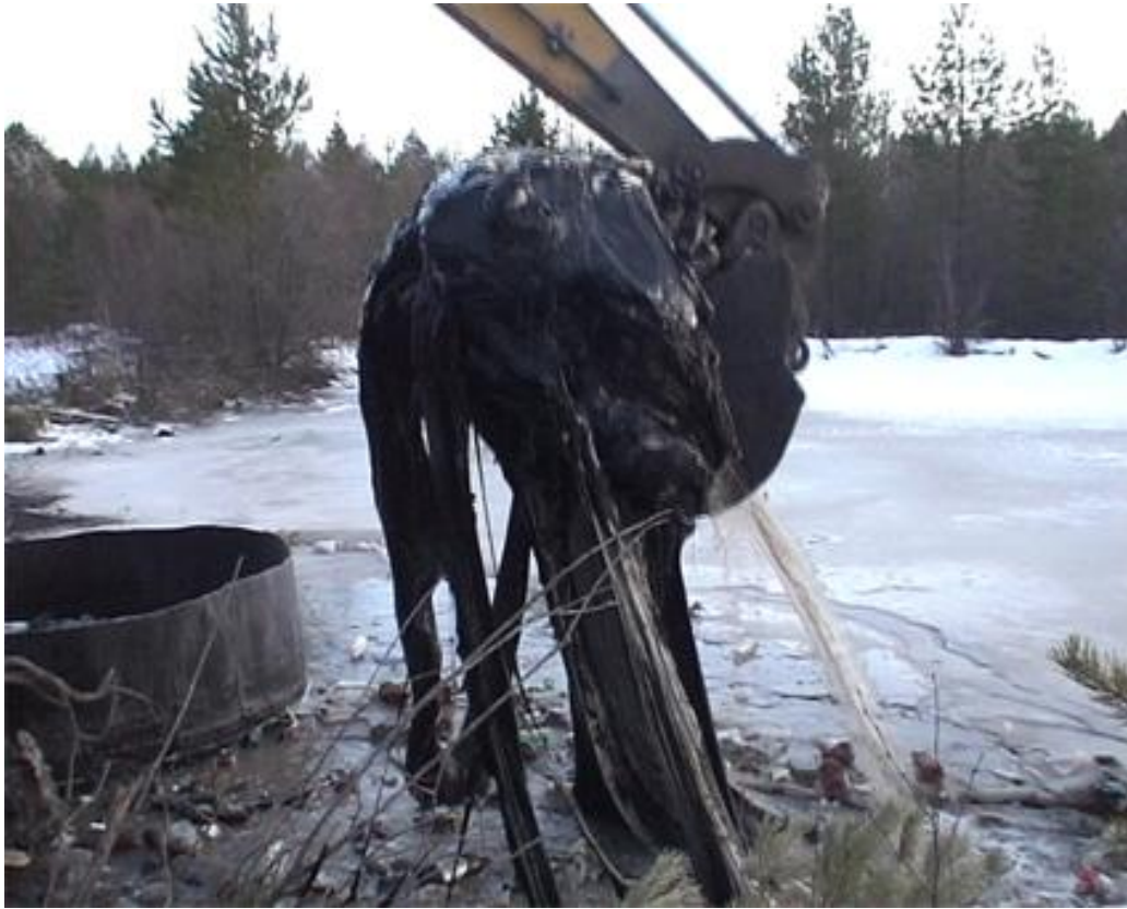
Figure 17. Collecting and Loading Oil Products from Oil Depot
