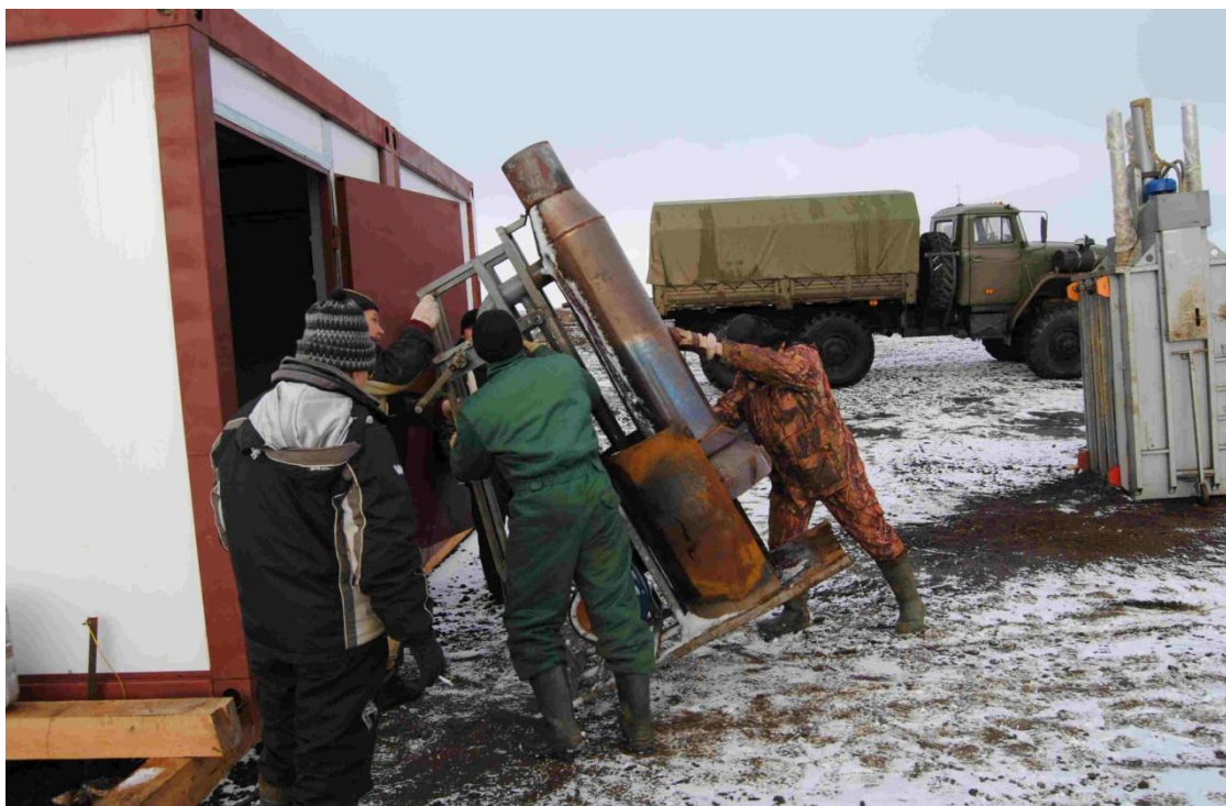
Figure 20. Installing Fuel Burnout Furnace and Steel Drum Compacting Press
