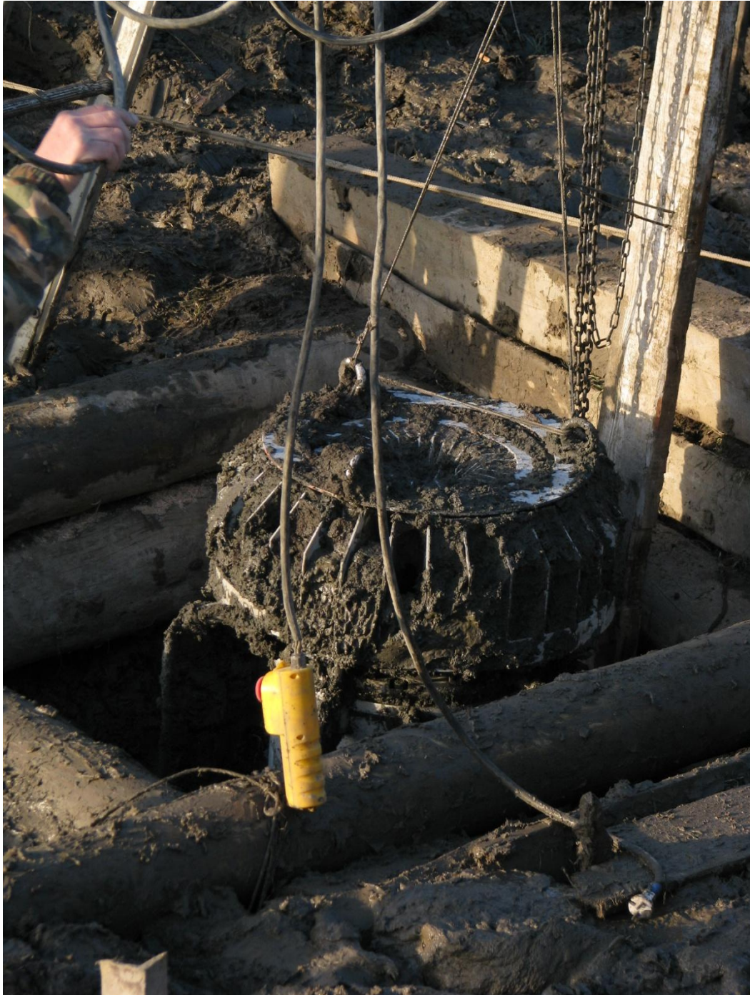
Figure 30. Removing RITEG from Thaw Sink
